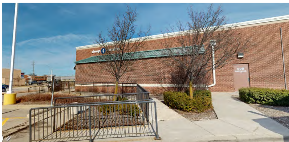
4 PHOTO OF EXISTING LANDSCAPE TO REMAIN - SOUTH SIDE
