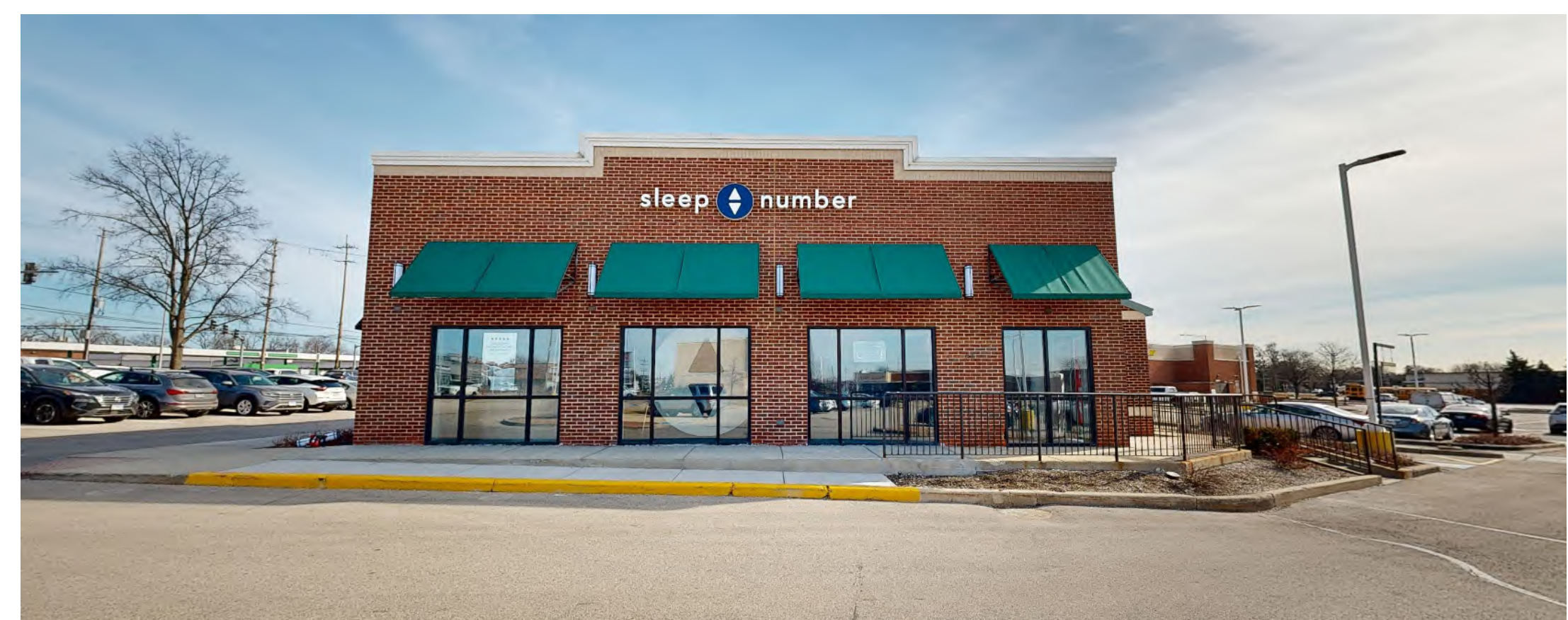
4 PHOTO OF EXISTING WEST ELEVATION
