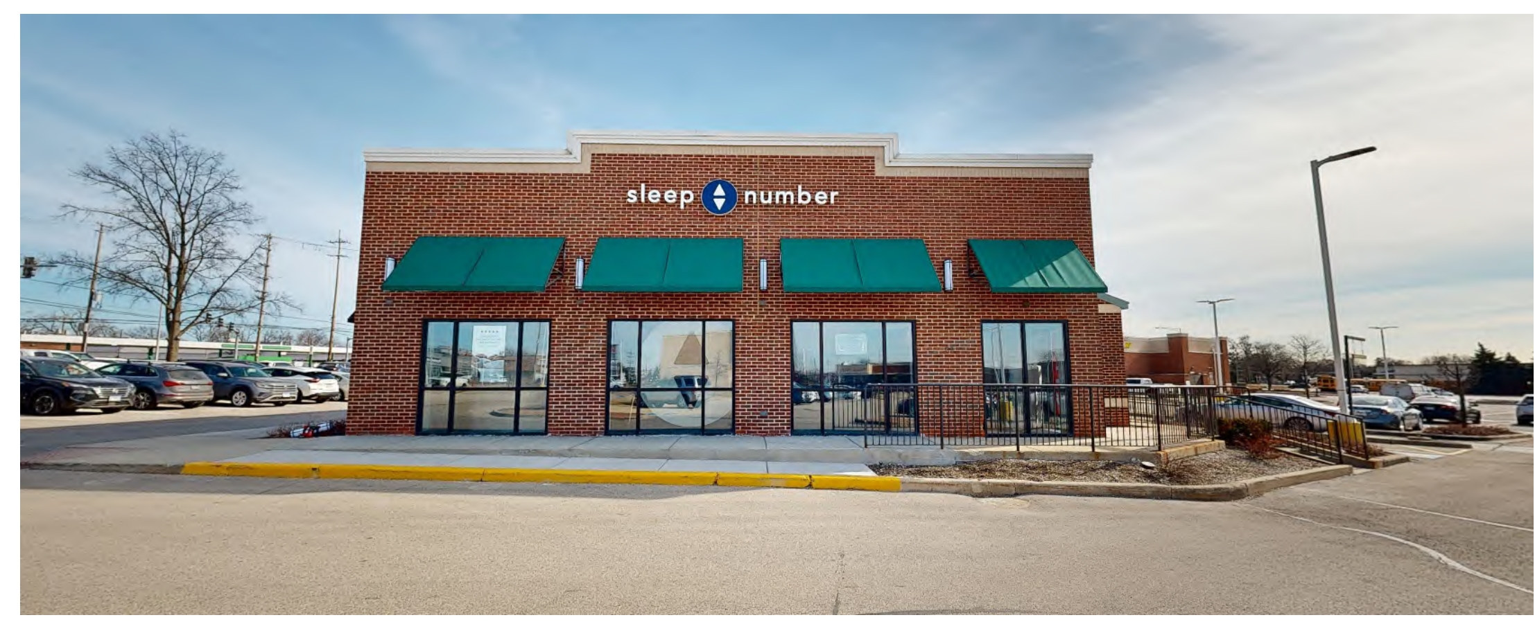
4 PHOTO OF EXISTING WEST ELEVATION
