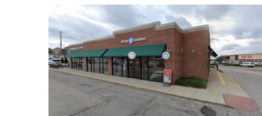
2 PHOTO OF EXISTING LANDSCAPE TO REMAIN - NORTH SIDE
