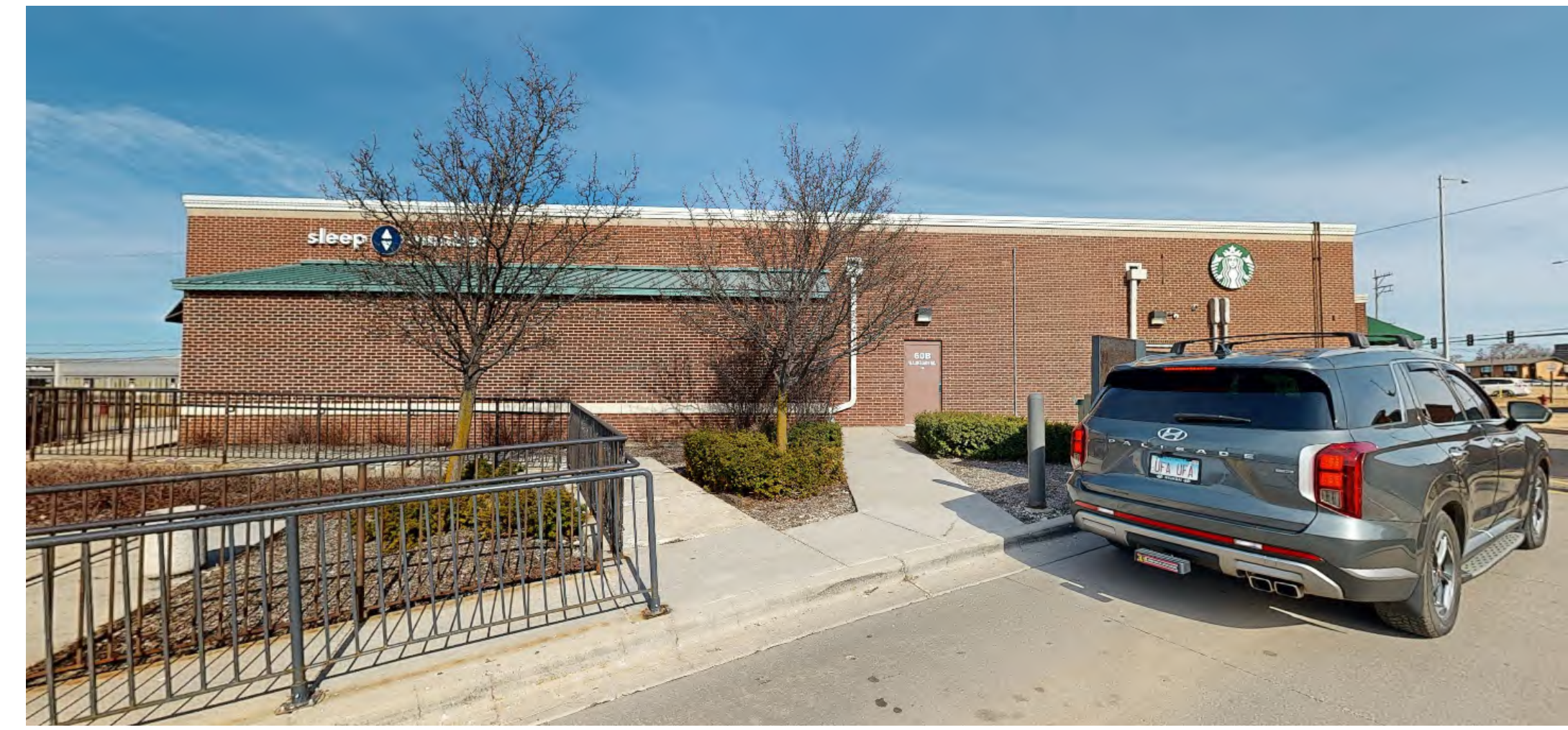
2 PHOTO OF EXISTING SOUTH ELEVATION
