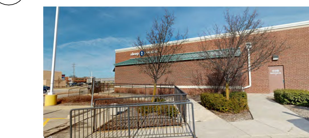
4 PHOTO OF EXISTING LANDSCAPE TO REMAIN - SOUTH SIDE
