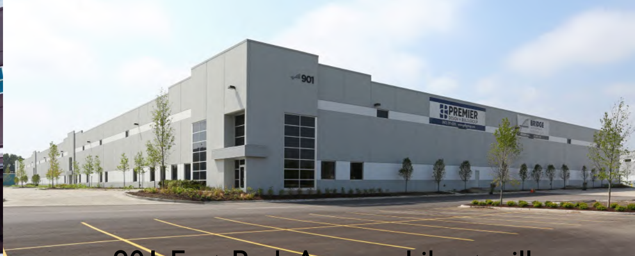
901 East Park Avenue, Libertyville
