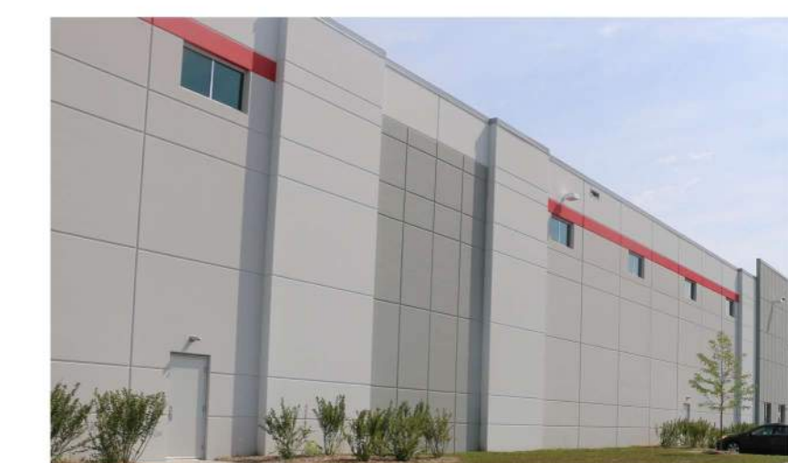
10 LAPPED PRECAST PANELS
