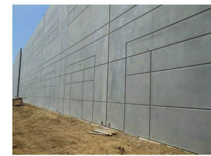
15 HORIZONTAL AND VERTICAL PRECAST REVEALS
