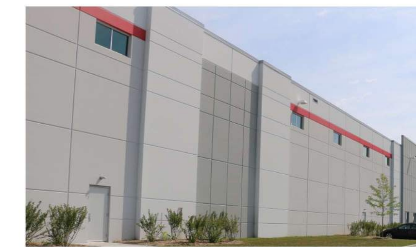
11 LAPPED PRECAST PANELS
