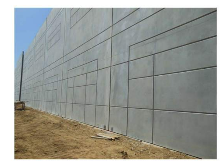
15 HORIZONTAL AND VERTICAL PRECAST REVEALS
