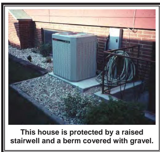
**Precautions:** The berm can only be built so high. It can be overtopped by a flood higher than expected. Being made of earth, it is susceptible to erosion from rain and floodwaters if not properly sloped and covered with grass and maintained. A berm can settle over time, lowering its protection level. The small floodwalls can crack and lose their watertight seals.
