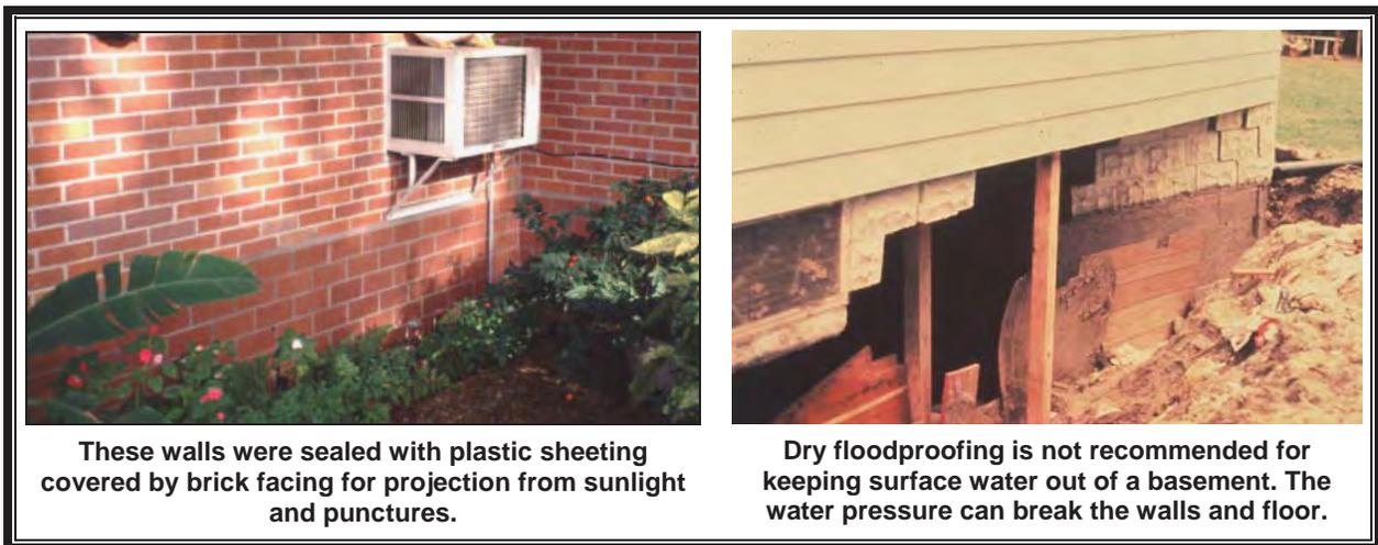
**Precautions:** It is very tempting for the owner of a dry floodproofed building to try to keep the flood out if floodwaters get deeper than two or three feet. This can result in collapsed walls, buckled floors, and danger to the occupants.
