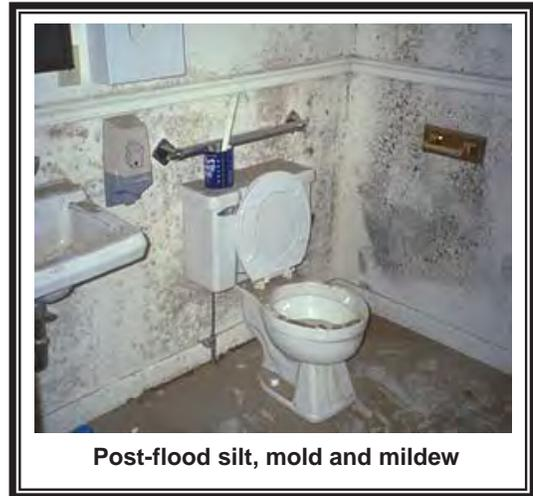
**Buildings:** Due to the relatively low velocities and shallow flood depths in the area, the most common type of building damage inflicted by a flood is caused by soaking. When soaked, many materials change their composition or shape. Wet wood will swell and, if dried too quickly, will crack, split or warp. Plywood can come apart. Gypsum wallboard will fall apart if it is bumped before drying out. The longer these materials are wet, the more moisture, sediment and pollutants they will absorb.
