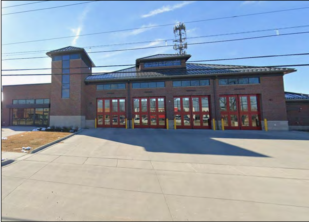
Elk Grove Village Fire Station
