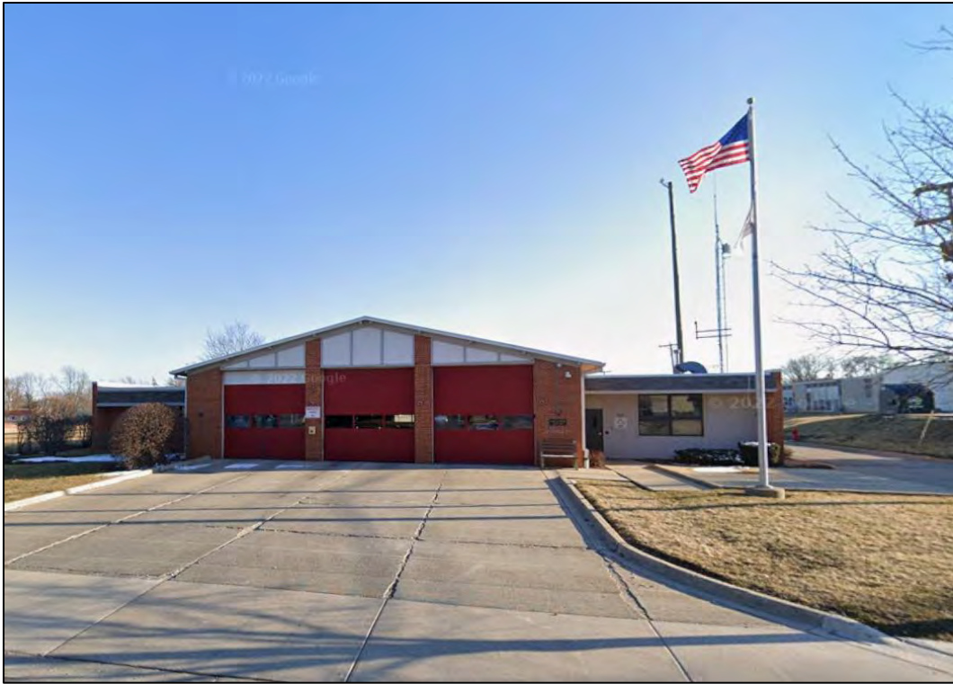
Hoffman Estates Fire Station
