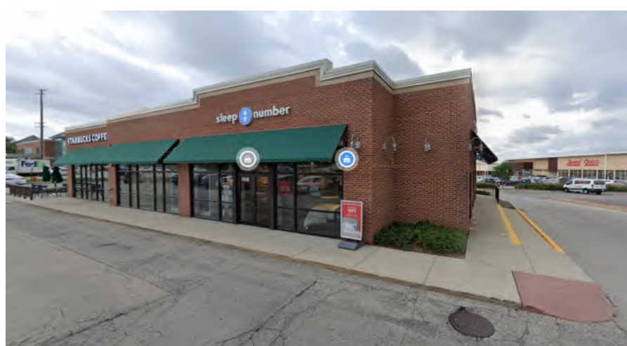
2 PHOTO OF EXISTING LANDSCAPE TO REMAIN - NORTH SIDE
