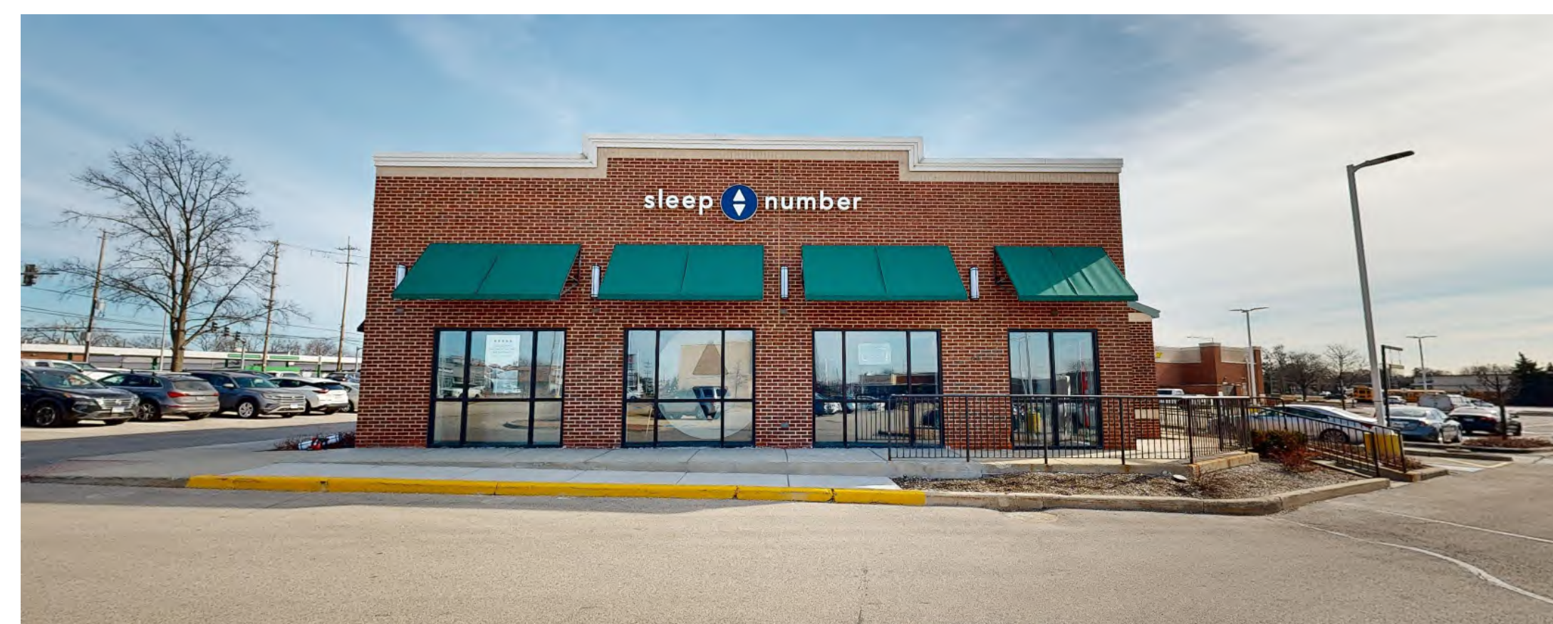
4 PHOTO OF EXISTING WEST ELEVATION
