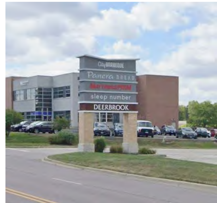
Existing faces to be removed & replaced
