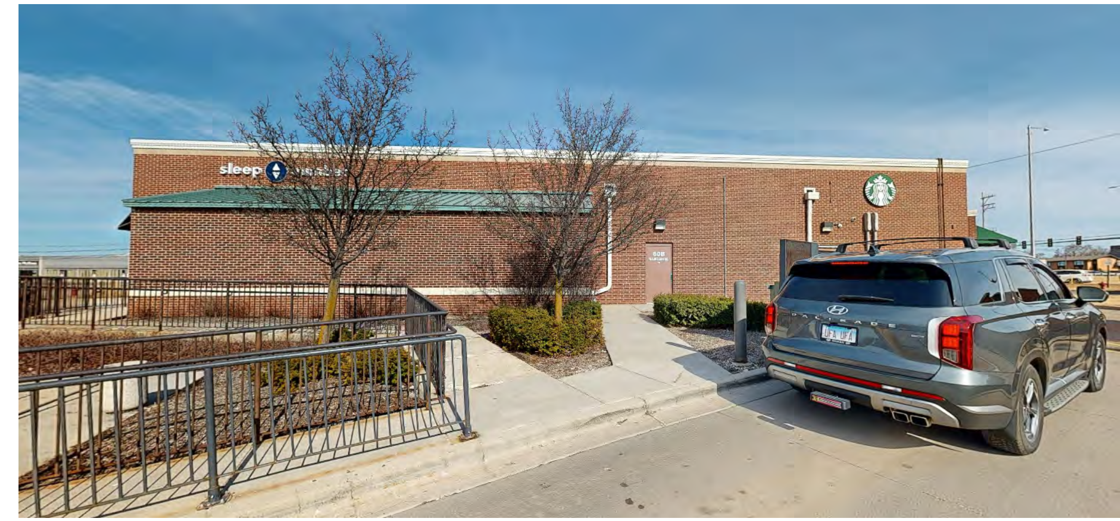
2 PHOTO OF EXISTING SOUTH ELEVATION
