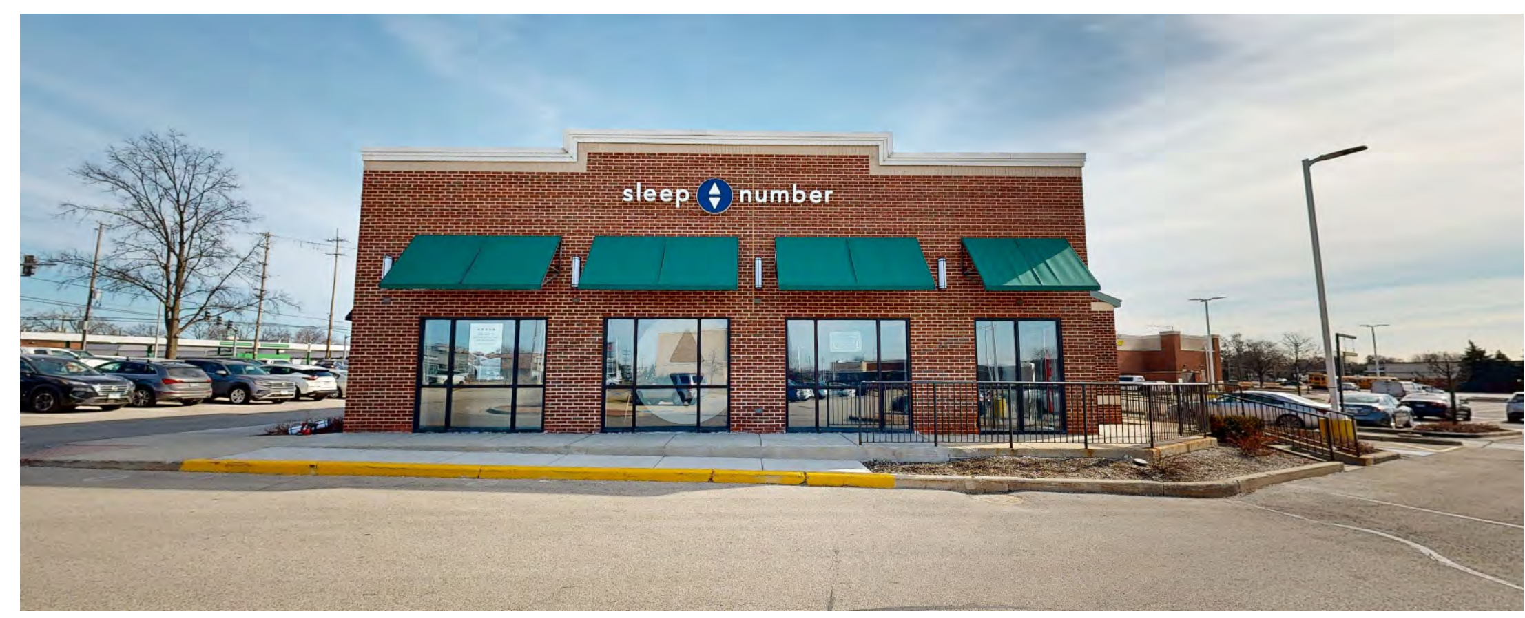
4 PHOTO OF EXISTING WEST ELEVATION
