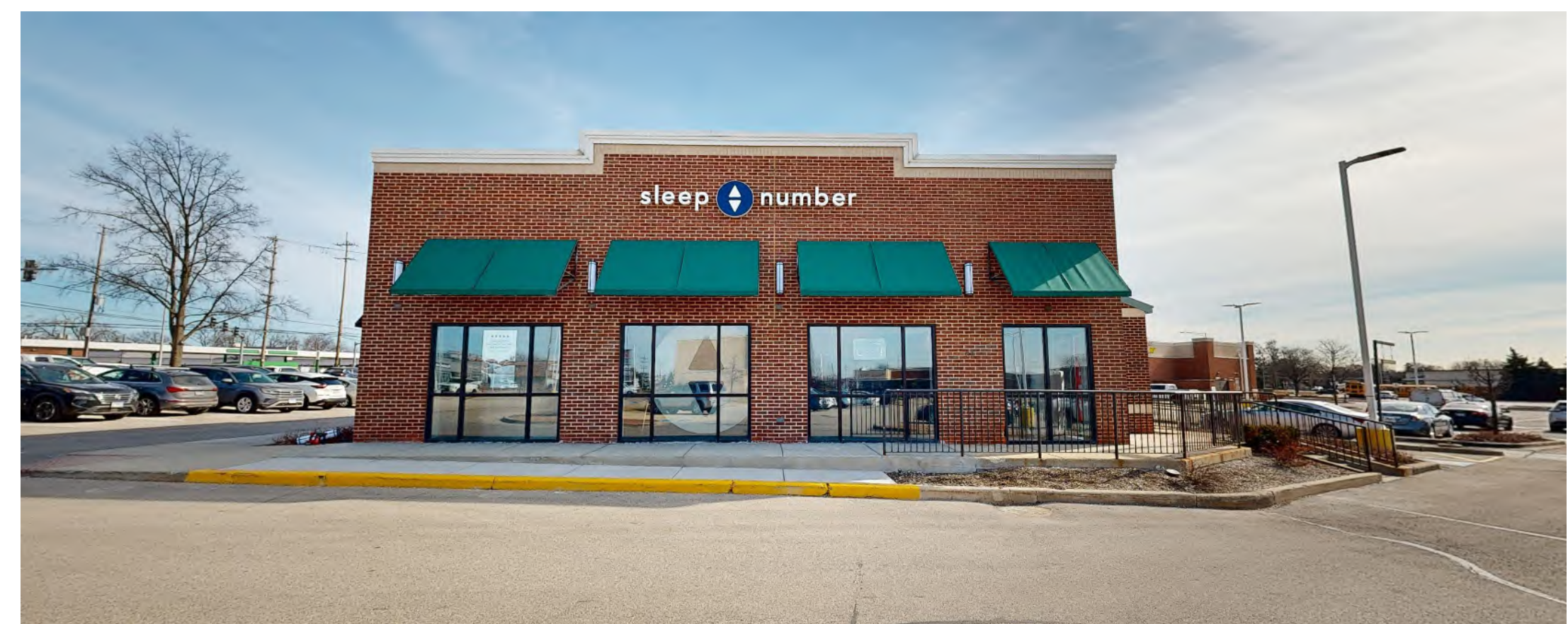
4 PHOTO OF EXISTING WEST ELEVATION
