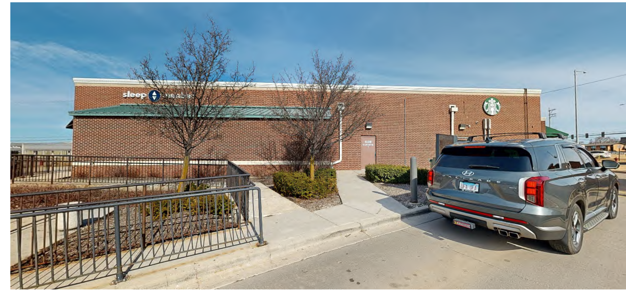
2 PHOTO OF EXISTING SOUTH ELEVATION
